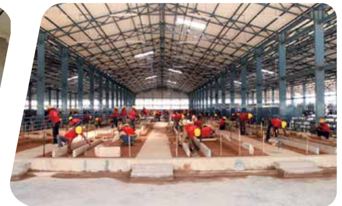
Pipe Fitter Training
